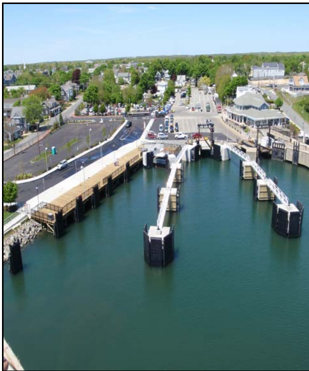
Figure 11. Completed Pier Facility at the Hyannis Terminal.
