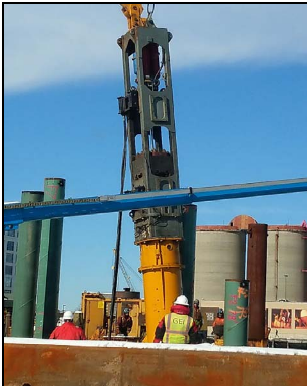
Figure 4 – Large Hydraulic Hammer – BSP CG240 - 176 kip-ft Rated Energy (photo courtesy of GTR)
