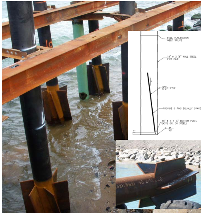
Figure 11a – Tapertube Pile SLT
