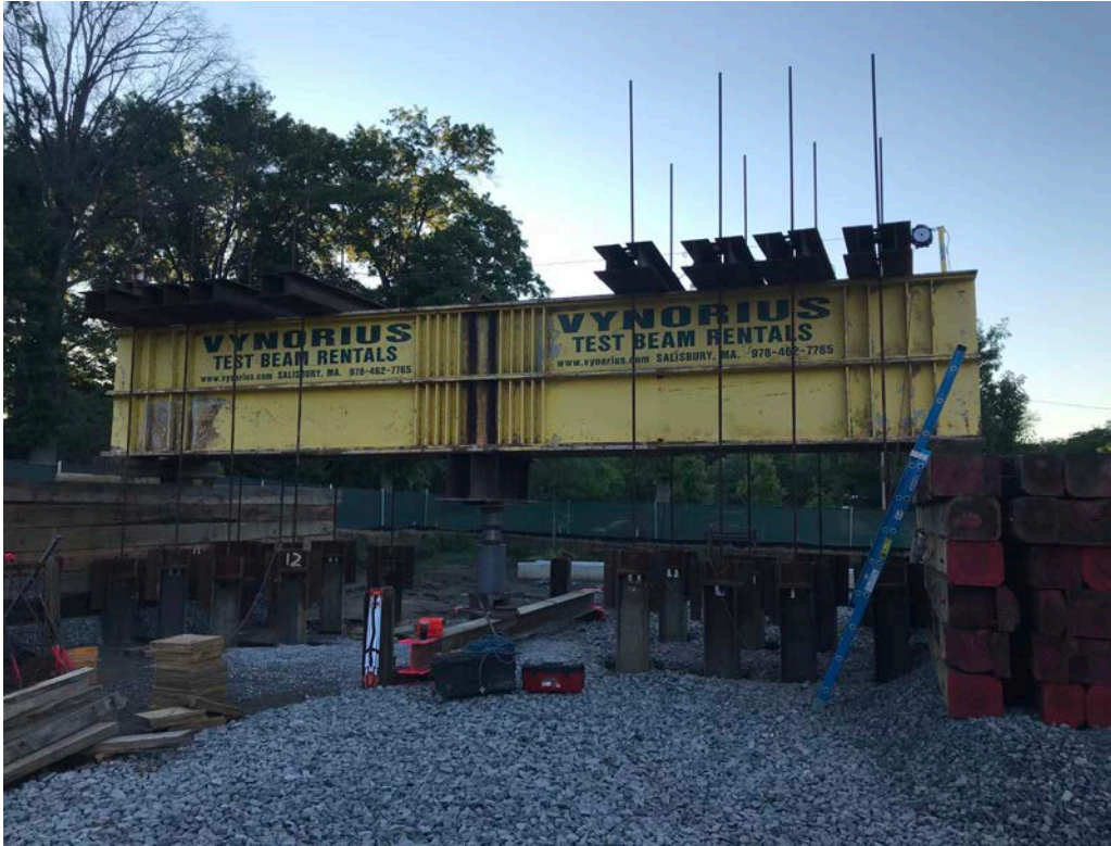
Figure 3 –Static Load Test Frame For Large Load
