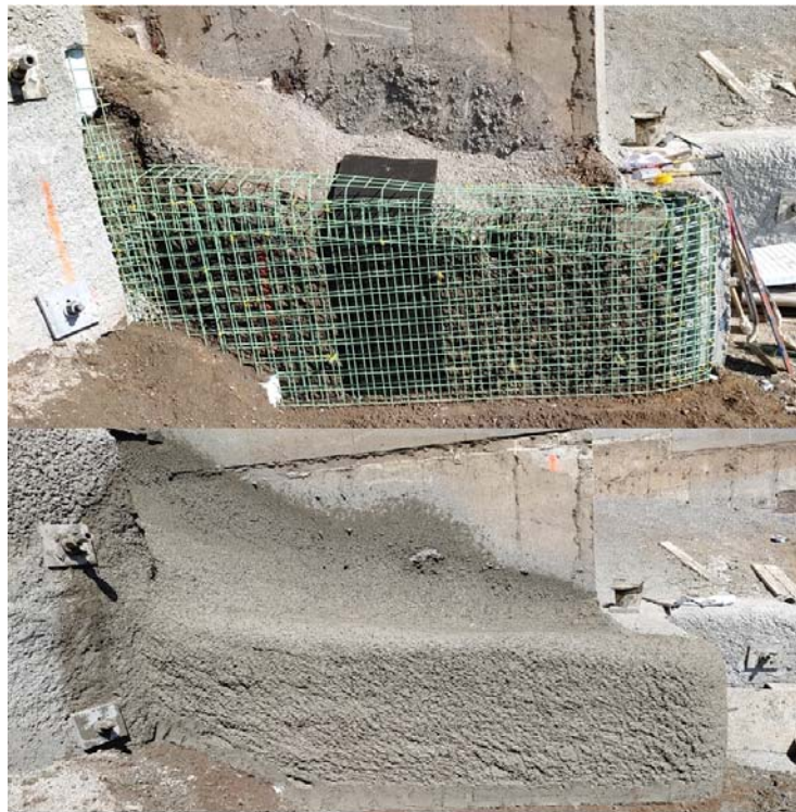
Figure 4: Shotcrete facing – rebar installation and shotcrete placement
