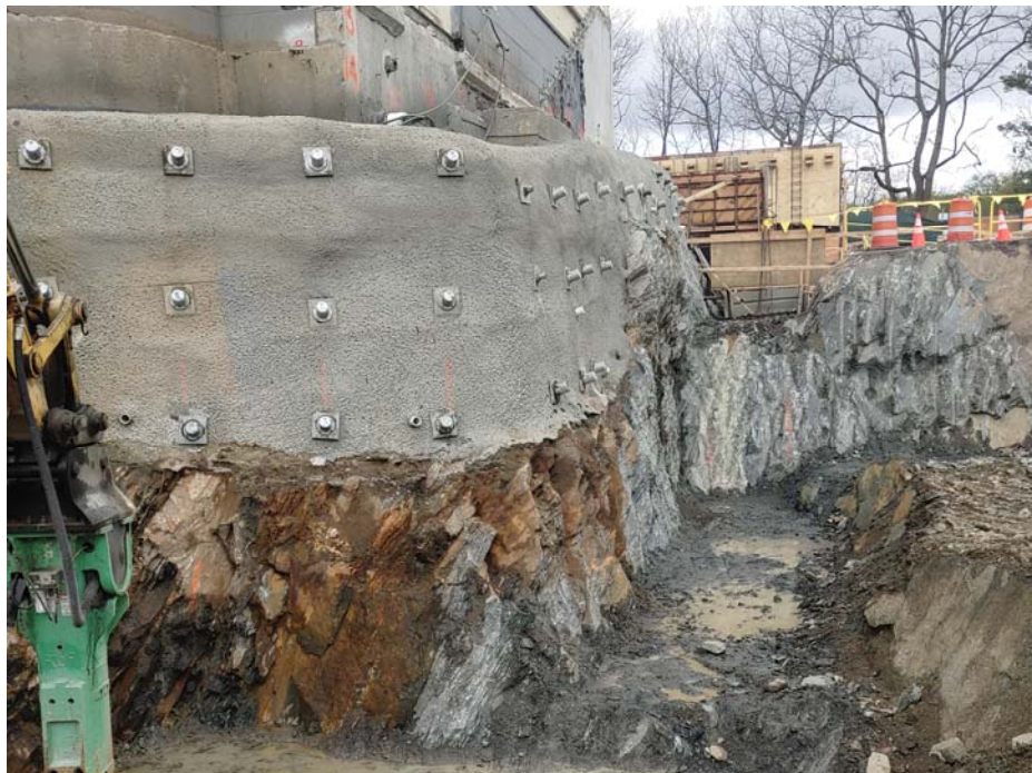
Figure 2: Photo of soil nail wall facing above excavated rock face.
